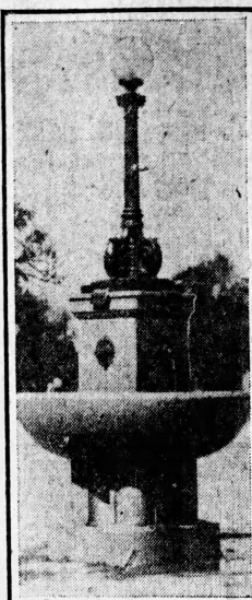
THE COMPLETED FOUNTAIN.
